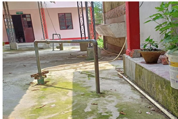
Submersible pumps for underground water
